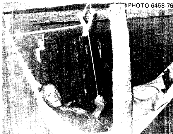
Fig. 4.10. Expedient bed-sheet hammock, useful to avoid severe shock effects in a shelter at high overpressure ranges. The man is operating an expedient shelter ventilating pump via an expedient pulley equivalent, a greased forked stick suspended on strings.
